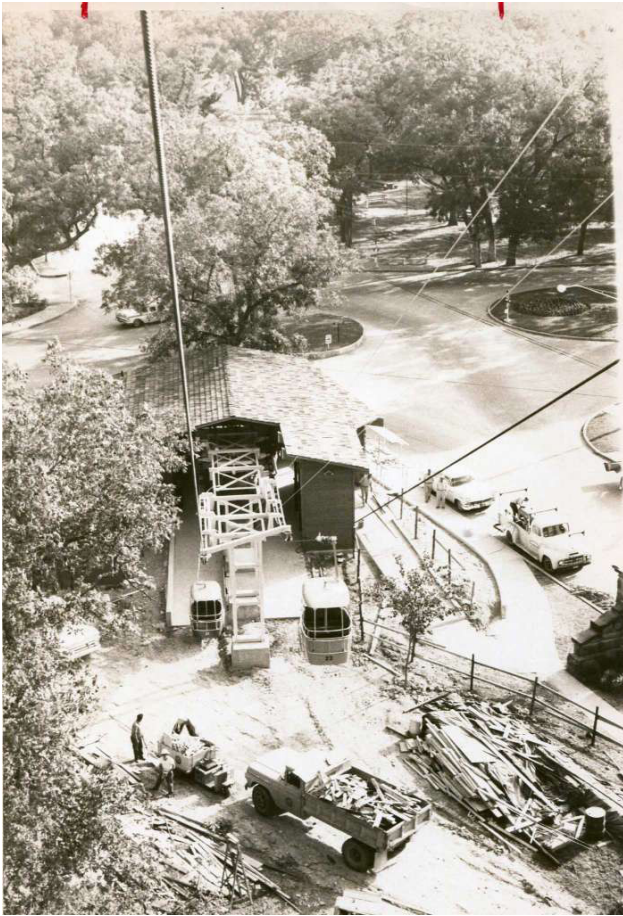
FIGURE 12-2. This image shows overhead portions of the HemisFair skyride in place, while construction continued on the infrastructure at the ground level. Source: Brackenridge Park Conservancy.
